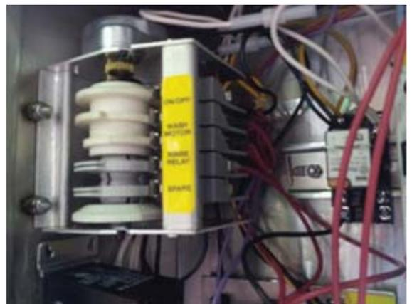
Cam timer with 3 fixed operational cams, 2 adjustable
