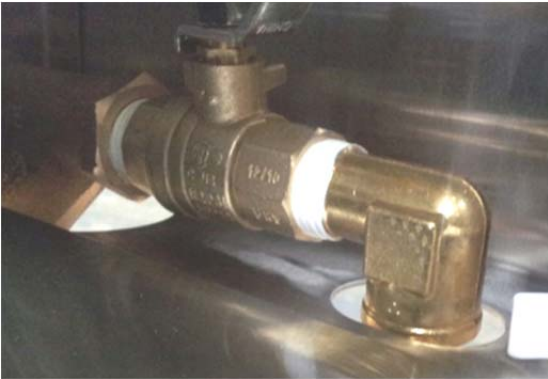
Drain hose connection to drain pipe
