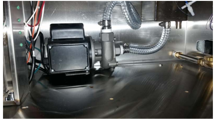
Wash pump with rinse pump removed
