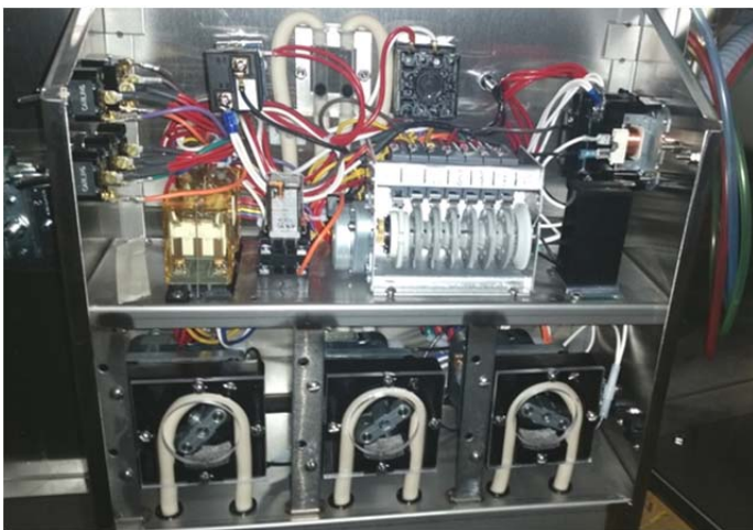
Showing deter, rinse, sanitizer internal chemical pumps
