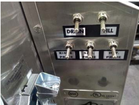
Showing controls on lower access door
