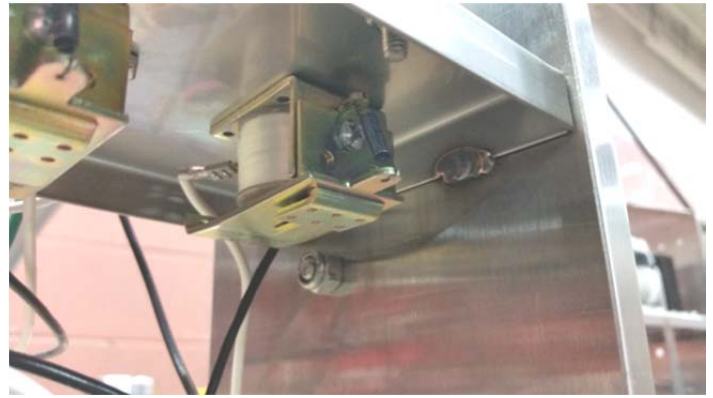
Optional buzzer for low chem alarm, under rack counter
