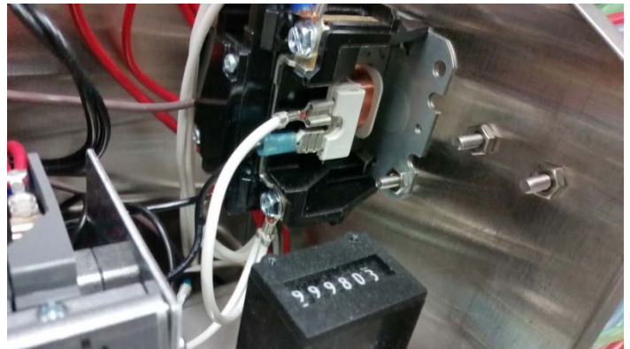
Wash motor contactor next to rack counter
