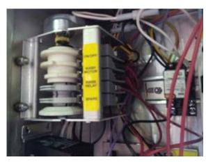
Cam timer with 3 fixed operational cams, 2 adjustable
