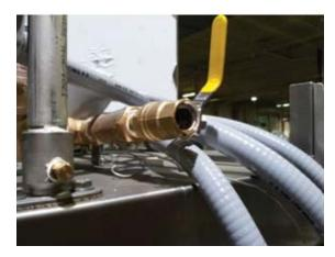
Showing final rinse mixing chamber, hot-water inlet to HT-25
