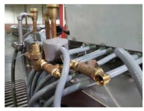
Hot water inlet manifold, single point ¾" pipe, PR valve
