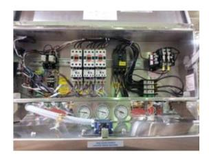
ADC-44 conveyor control box for 3-phase power
