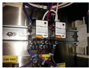
Conveyor motor control relays
