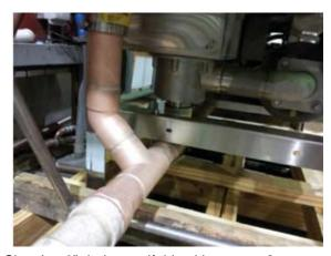
Showing 2" drain manifold exiting sump & scrap box
