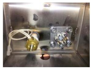
Showing thermostat and sustainer heater terminals\*
