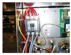
Showing booster contactor, yellow signal wire
