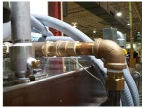
HT hot water inlet ball valve, connected to booster line
