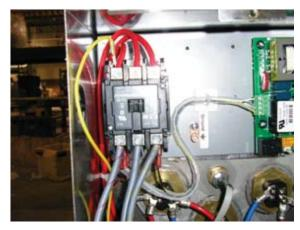
Showing booster contactor, yellow signal wire
